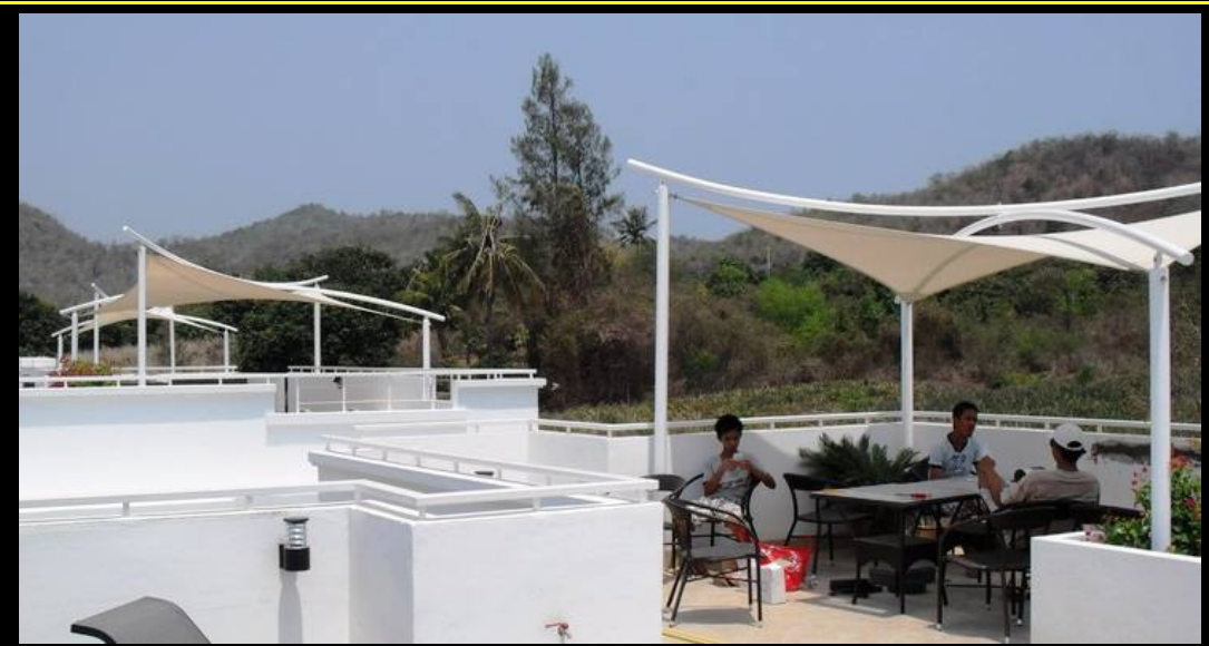
Roof-top shade structures Oriental Mountain View, Hua Hin
