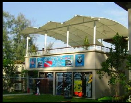
Restaurant roofing Dewa Resort, Naiyang Beach, Phuket
